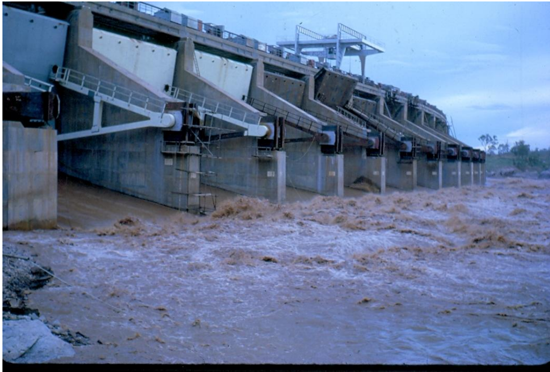
The Dam passes the 1962-63 flood
