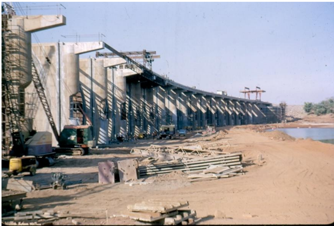
The Dam nears completion... all piers to full height... the roadway approaches the western abutment.
